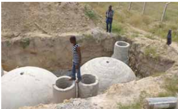
Biogas vergister in aanleg in Accra, Ghana
